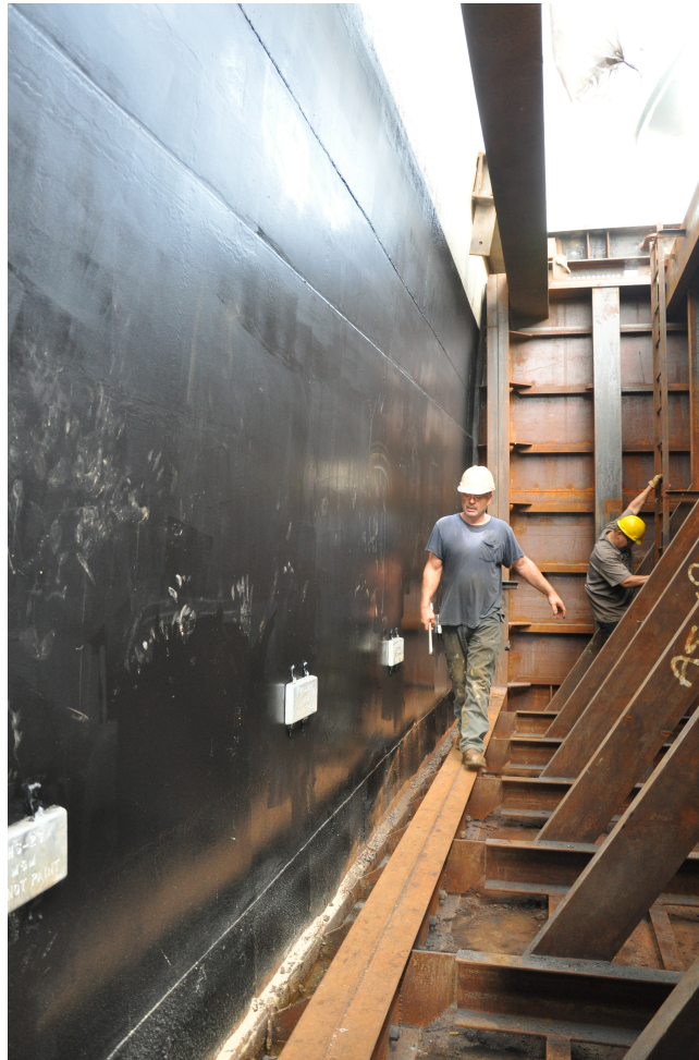
Figure 12. Final Exterior Product with Zinc Anodes
