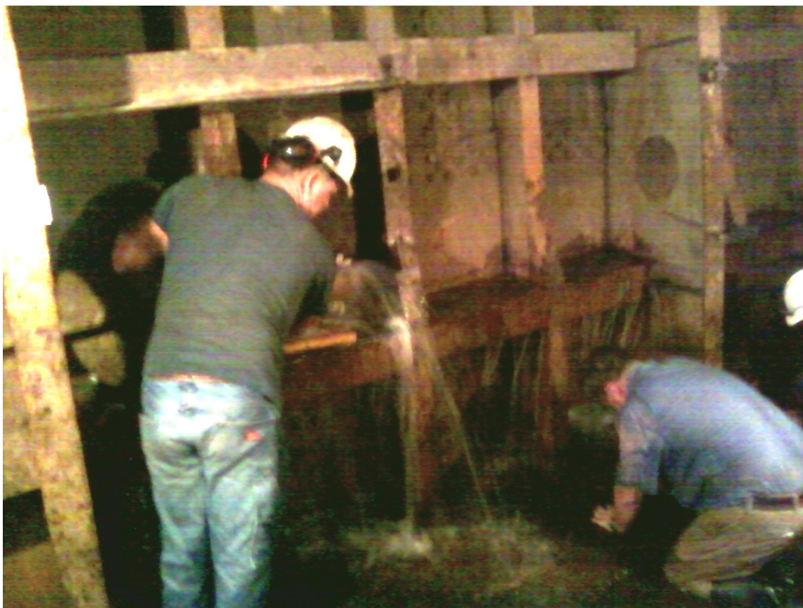
Figure 11. Patching a New Leak
