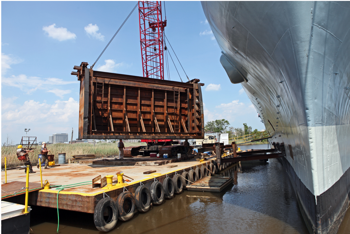
Figure 2. Cofferdam Installation
