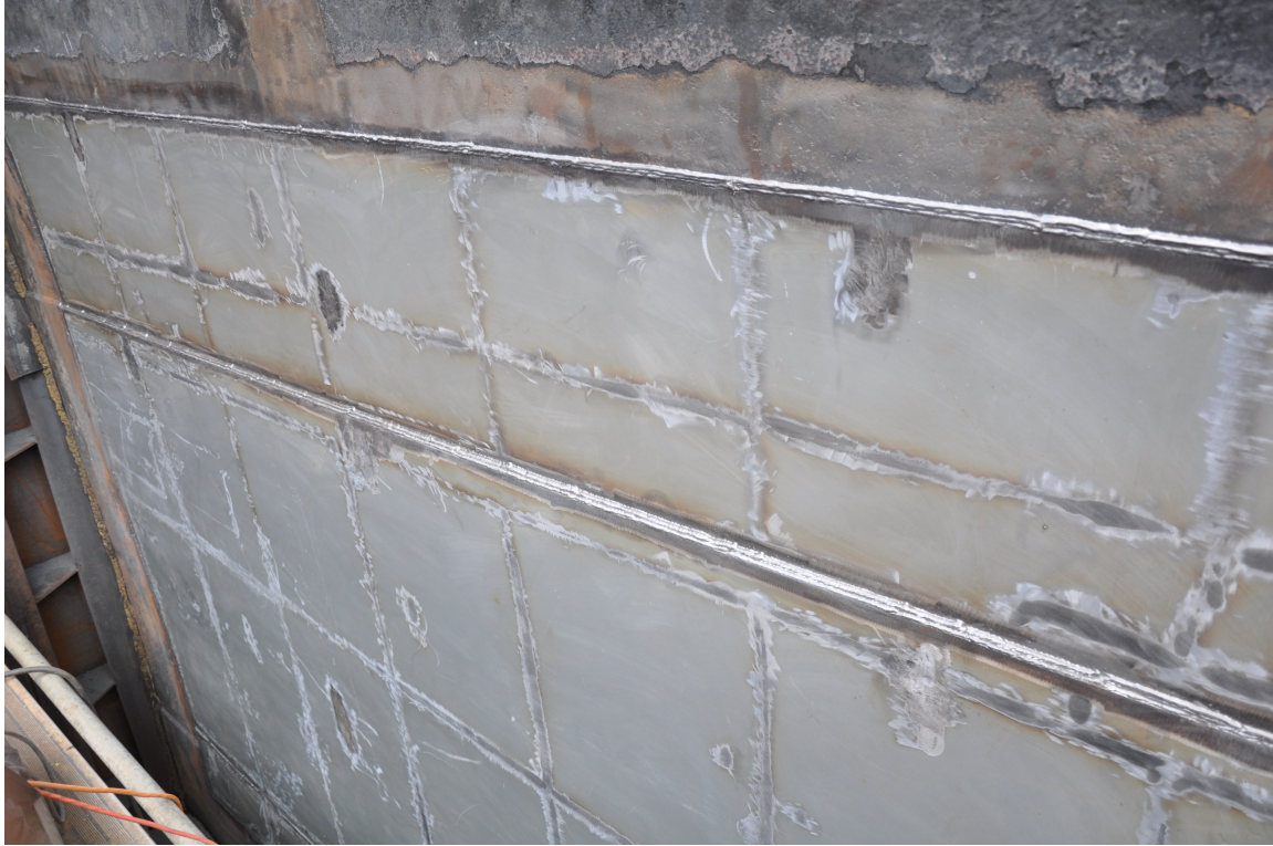
Figure 10. New Plating Installed
