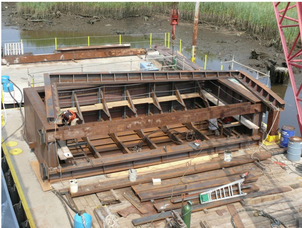
Figure 5. Cofferdam Flanged Seal Face
